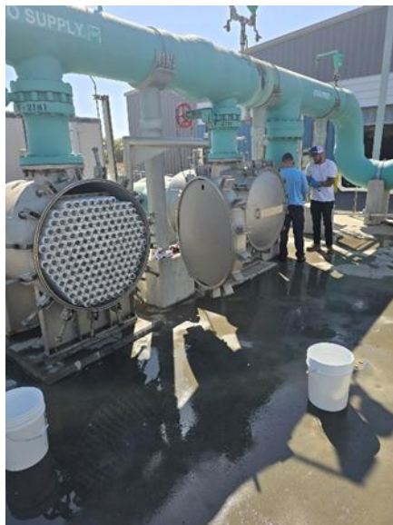
Staff replacing cartridge filter
